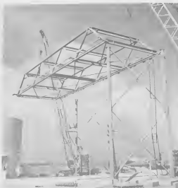
THE FOURTEEN-ton truss section of Lago's new pipe bridge was erected by the contractor March 19 with the aid of Lago's two heavy-duty cranes. Forty-foot columns support the section. E SECTION di aguanté di dies-cuatro ton na e brug nobo di tubo na Lago a wordé crui door di e contratista Maart 19 cu ayudo di dos grusaan piá di Lago. Columnanan di cuarenta pia ta wanta e seccion.
